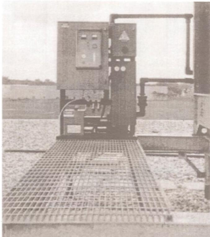
**Fig. 1. Typical Cooling Tower Ozone Generation System**
