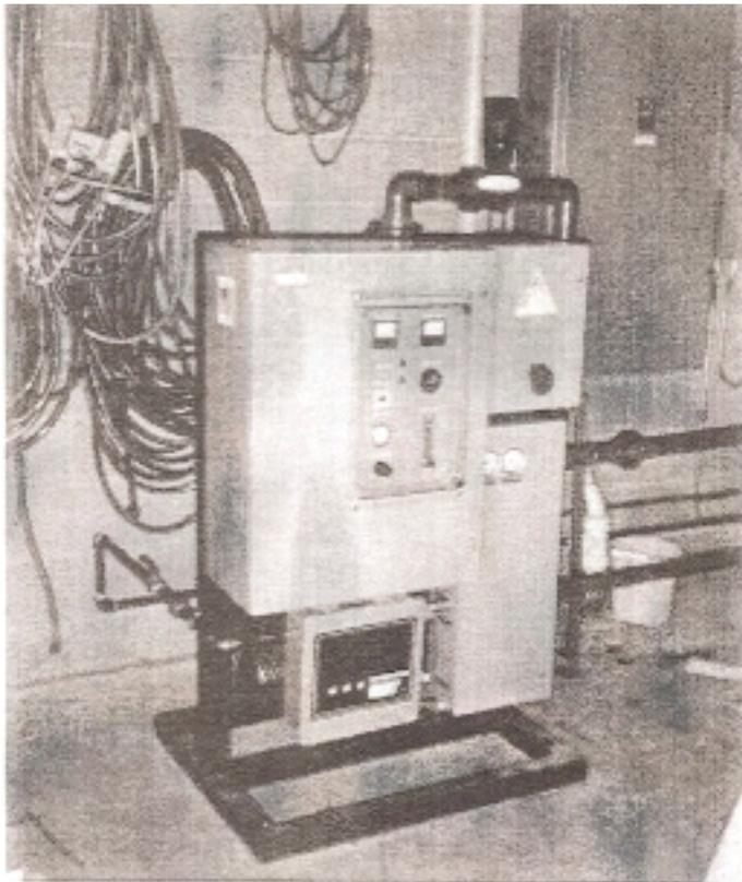
**Fig. 5. Ozone System, Showing Piping and Skids**
